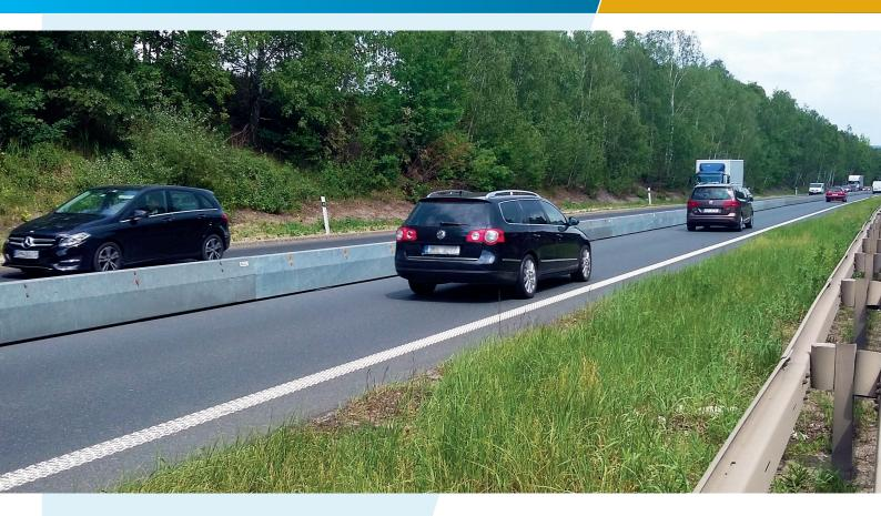
T3 barriers are used for creating temporary traffic lanes. The narrow design ensures that as much of the carriageway as possible is available to traffic. The T3 barriers have been tested in compliance with EN 1317-2.
